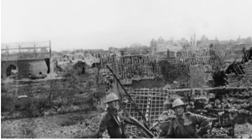
Shattered buildings in the French village of Lagnicourt, which was captured by the Australians in late March 1917 as the Germans withdrew towards the Hindenburg Line. The Germans heavily shelled the village as they retreated.
